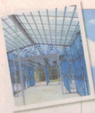
The steel frame takes shape
